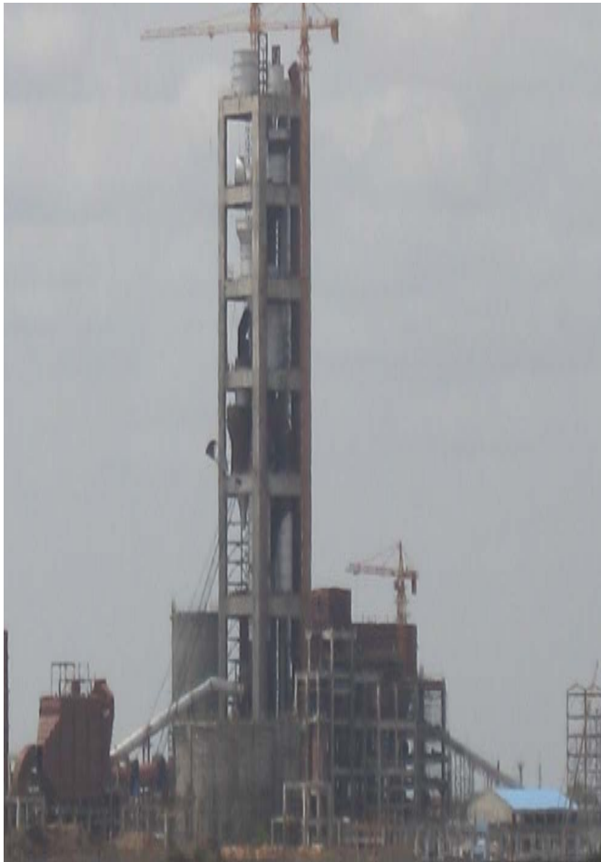
Kadapa, AP Cement Plant
