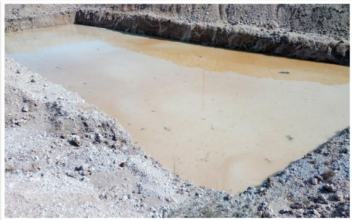
Water Harvesting Pond at Kallakudi Village
