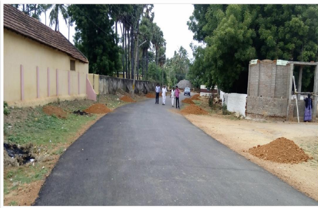
New Road Laid At Temple Car Street At Vadugarpet Village
