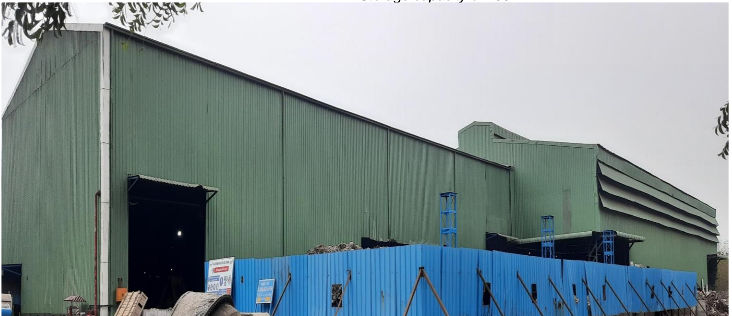
Newly Constructed Shed for Handling AFR materials
