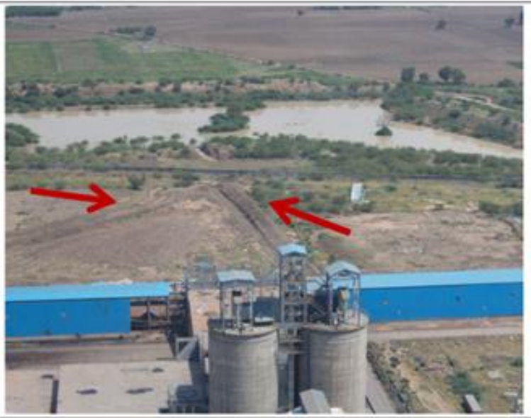
Storm Water Drains connected to Pond
