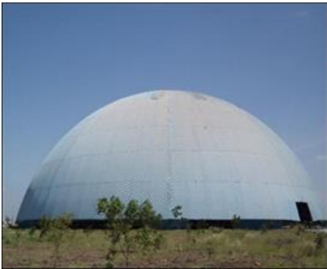
Lime Stone Storage Shed
