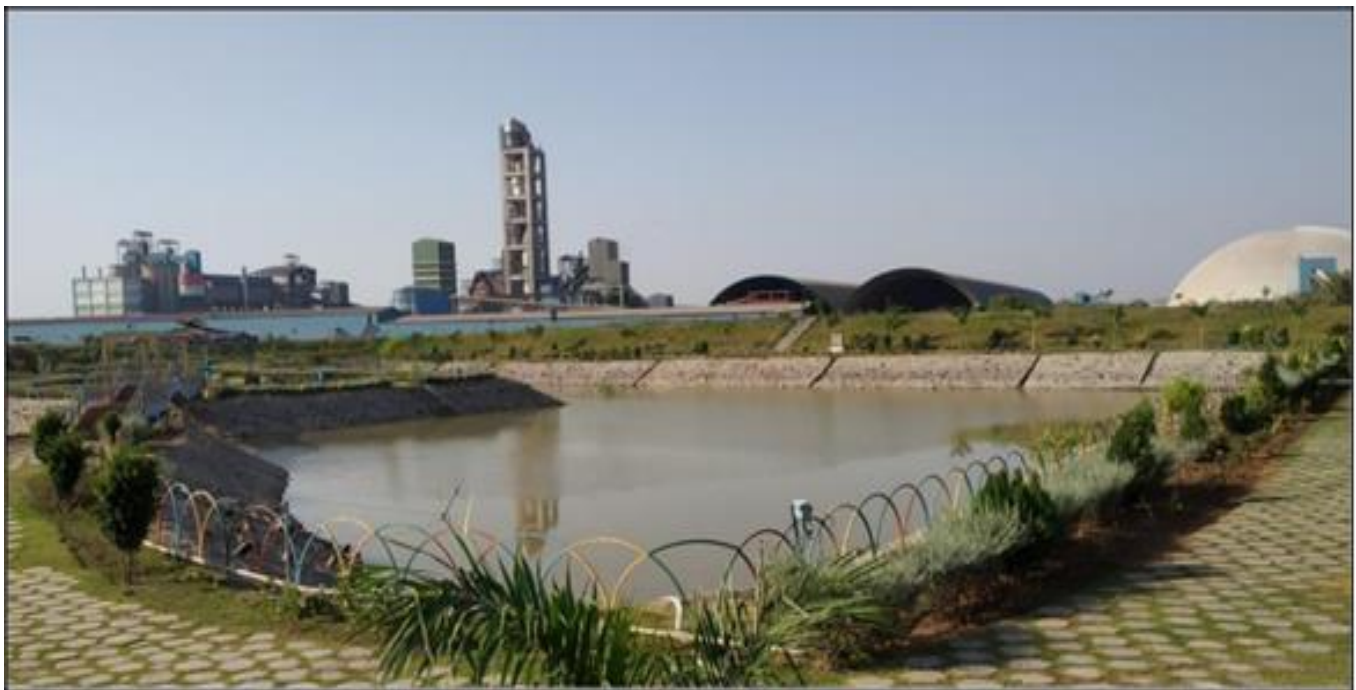
Plant inside Rain Water Harvesting Pond
