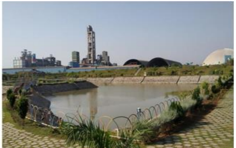
Plant Rain Water Harvesting Pond
