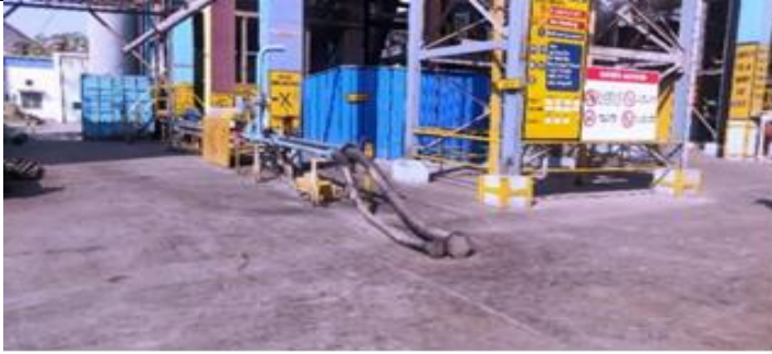
Pneumatic System available for unloading and feeding of Carbon black powder to the mill through
