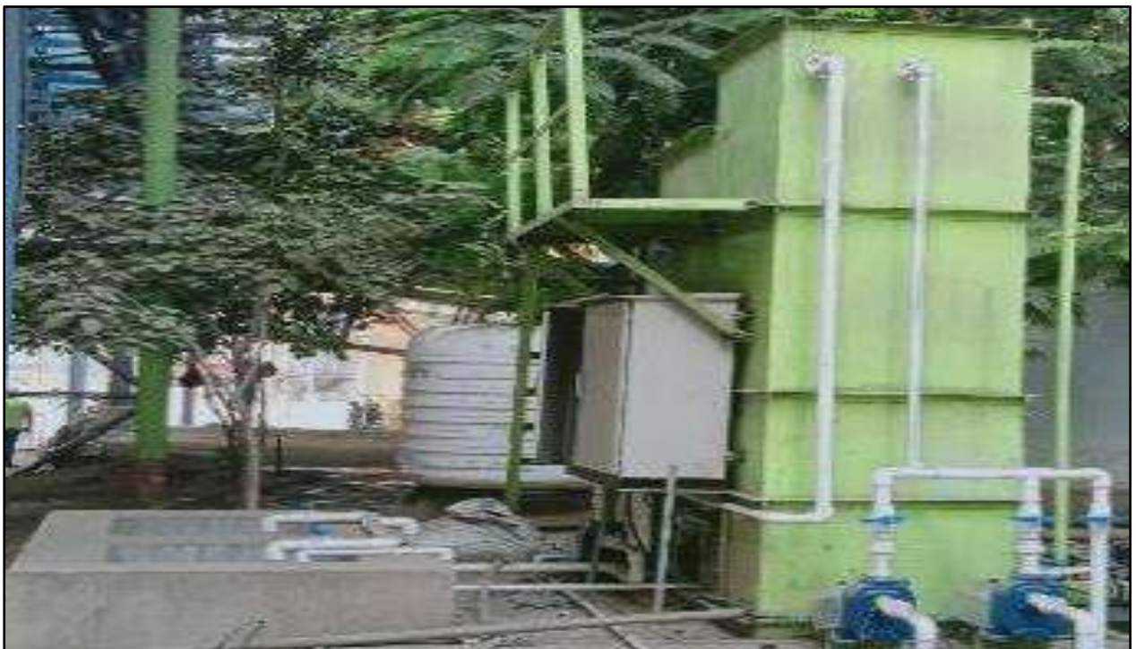
Sewage Treatment Plant Installed at CCR Area
