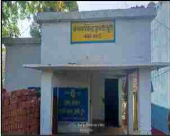
Renovation of Aganwadi
