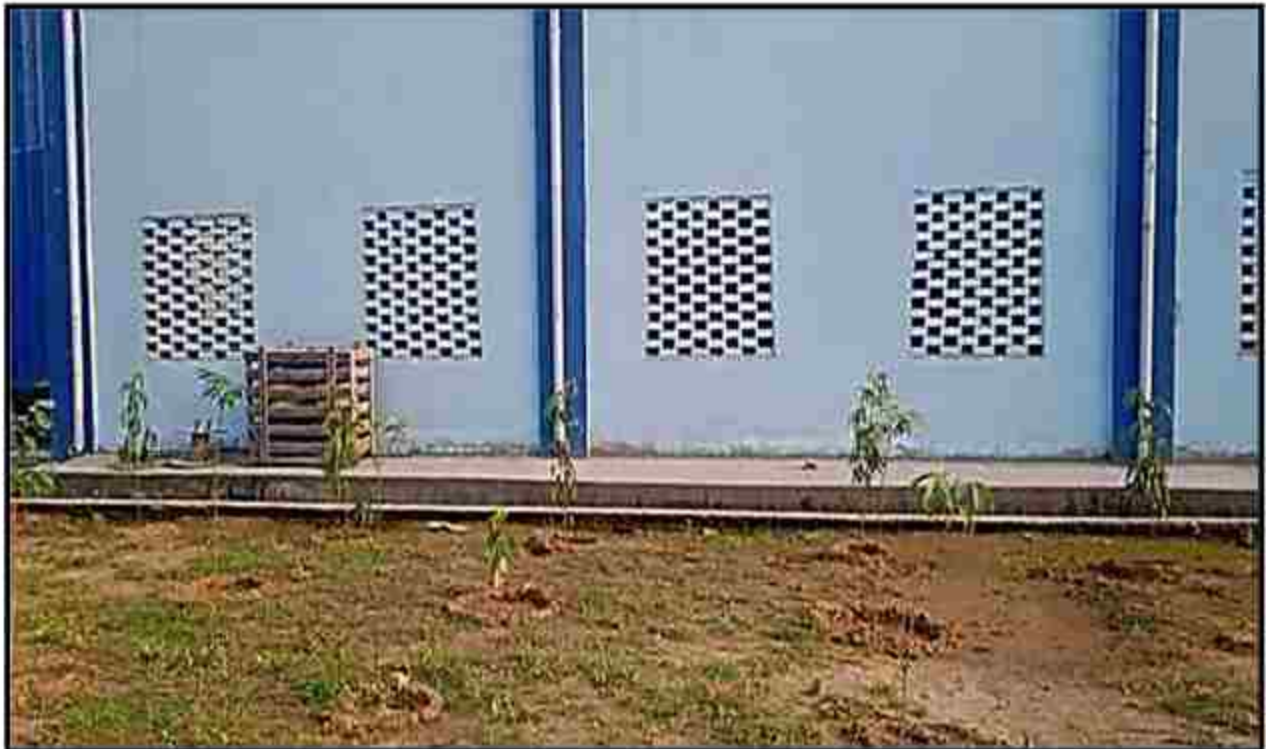
Rooftop Rain water collection pipe line, concreted drain connected to recharge pit near Packing plant building
