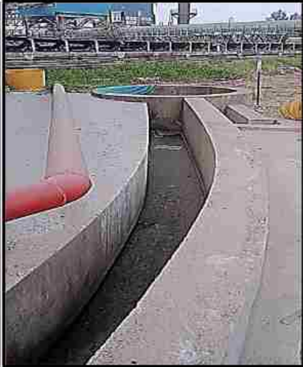
Connecting drain to Rain water Harvesting recharge pit near stacker reclaimer
