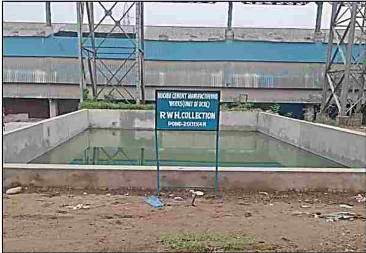
Rain Water collection Pond constructed Capacity: 925 KL
