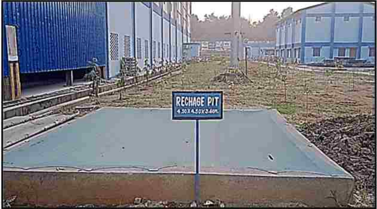
Rain water harvesting recharge pit near Packing plant
