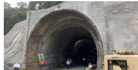
Sevoke-Rangpo Railway Tunnel, Sikkim Blended Cement in Concrete Tunnel Lining
