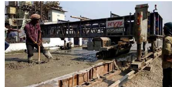
NHAI Project, Bihar & West Bengal Blended Cement usage in Pavement Quality Concrete
